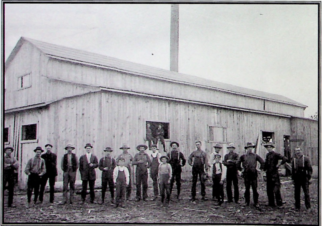
Stave Factory early 1900s
