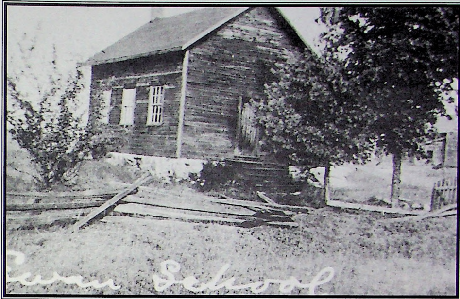
The Ewan School SS #6 was located on Lot 30, concession 15. Settlers were never very numerous and the school was closed by 1915. However, church services continued to be held there. Due to the remote location the congregation usually represented at least 3 or 4 different denominations. The Ewan settlement was not known for the quality of farmland and was used more for cattle ranching. Families came and went, but the White and Jackson Families remained over the years.
