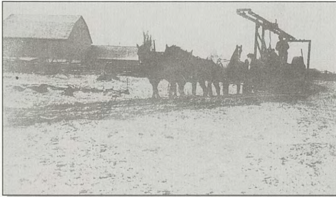
Will Rettie drawing the drilling machine used to make the holes for dynamite, from the road into the quarry [Joe Rettie]
