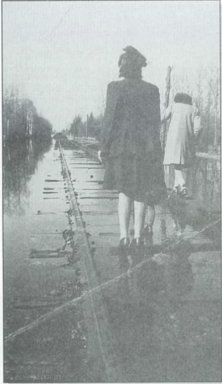
The 1946 spring flood, looking south-west along the railway tracks, behind Wright's Store in Burnt River [Lorna Sheehey]
