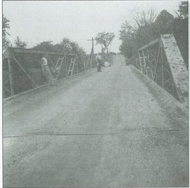
Charles O. Hodgson, standing on the old East Line bridge over the river, 1952 [Bernice Hodgson]
