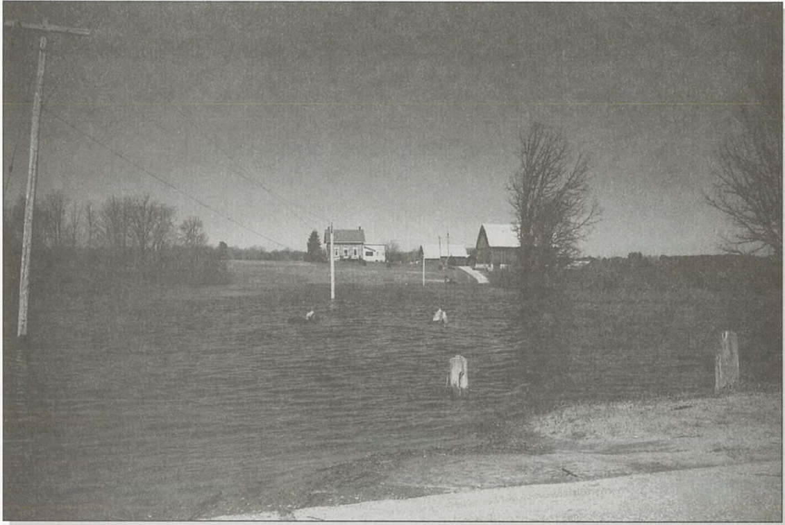
The roadway and bridge to the Armstrong farm, completely cut off during the flood of 1991 [Bernice Hodgson]
