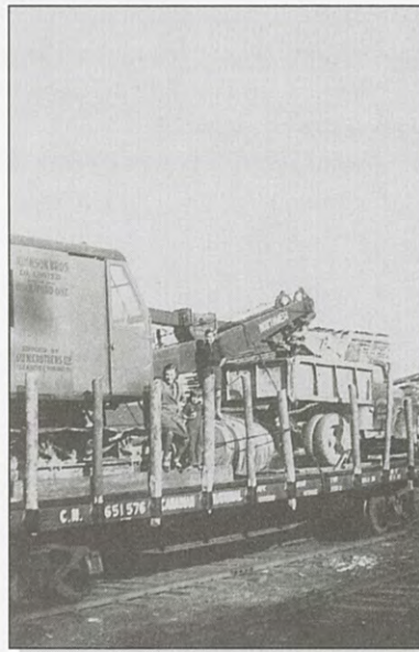
A shovel, truck and dragline, from the road construction on the bi-pass, being loaded at the Burnt River Station in 1938, for shipping to next construction site at Lake Nipigon [Lorna Sheehey]
