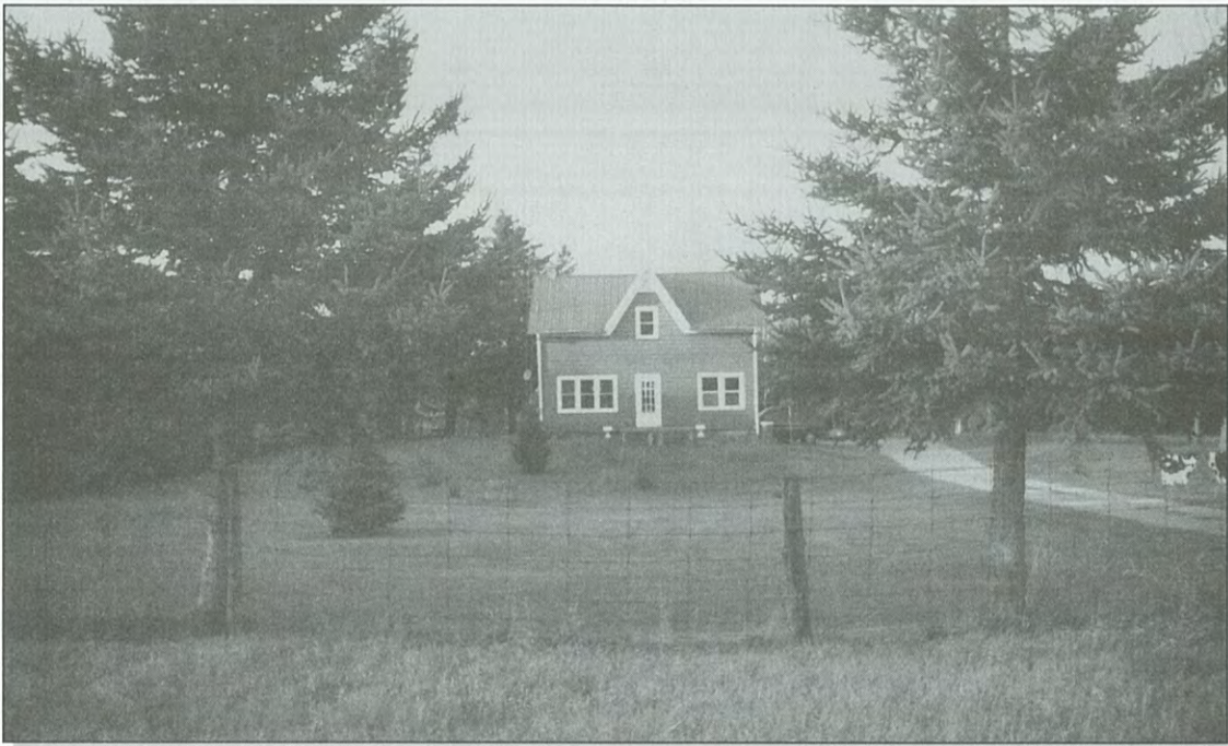
The house built for Rol and Minnie Young at 3003 County Rd. 121.
