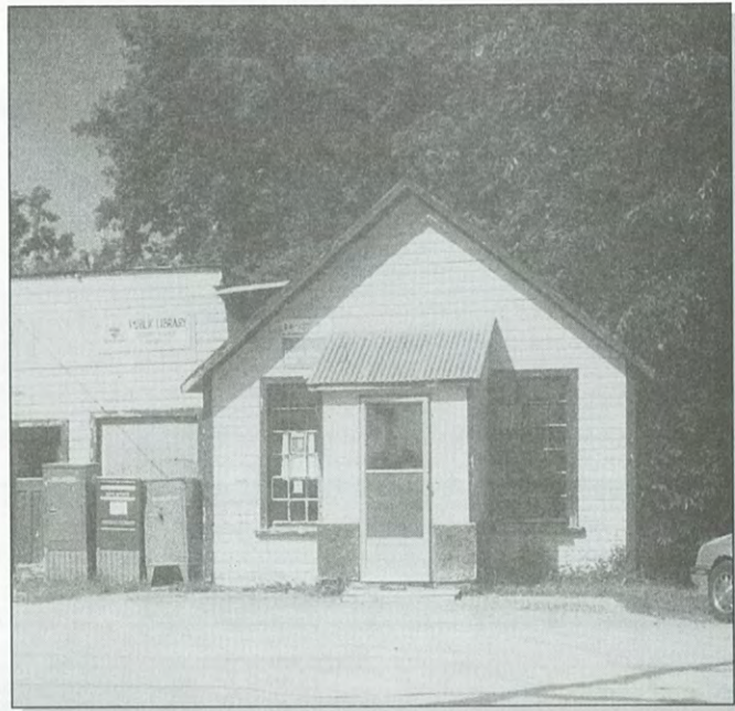
From April 1, 1970, until July 1, 1993, the Burnt River Post Office, and with its commencement in February 1973, the Burnt River Library, were housed in this small building beside the General Store, which was owned by Roddie and Eva Wright. Both were operated in this period by Mrs. June Hunter, as Postmaster and Branch Librarian. [June Hunter]
