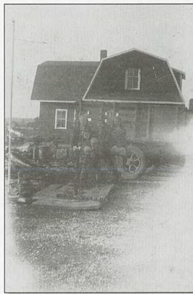
The Morgan House the day after the Burnt River Village fire, 1944 [Marg Sheehy]
