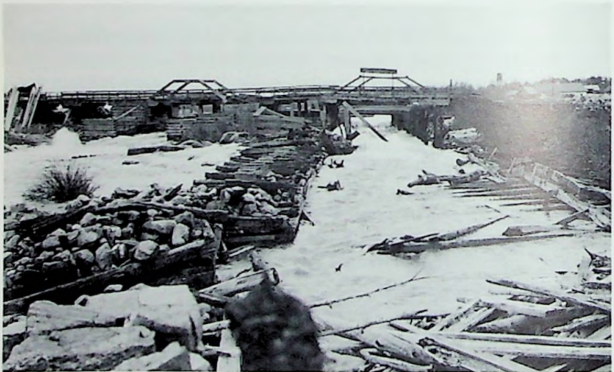
Buckhorn dam and bridge. N.B. Two chutes ( centre ). Lumber being used during construction of new dam ( left ); Buckhorn Cheese Factory ( right background ) and tower for whey delivery to Piggery Bay ( left of factory ). (Courtesy Trent-Severn Waterway).
