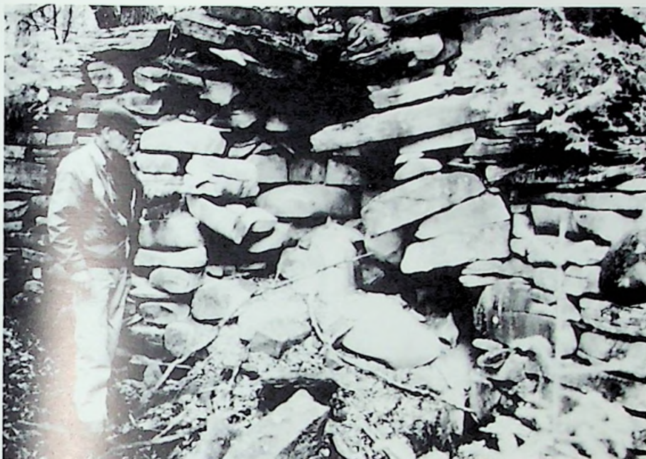
Art Parker examines lime-kiln remains on his parents' former farm. N.B. Made of interlocking slabs of local limestone, without mortar, the kiln enclosed a central cavity in which pieces of limestone were heated from below and ventilated by the chimney above. After several days the burned limestone was slaked with water and the lime used in building-mortar. (Courtesy Alan Brunger).
