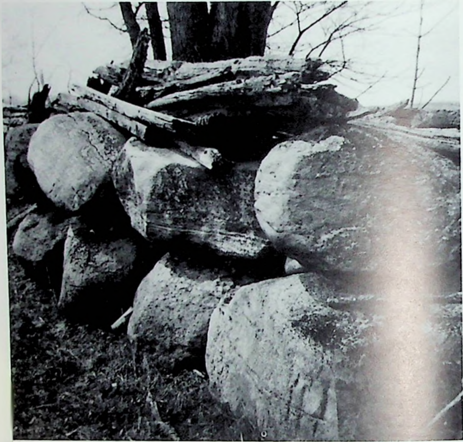
Fence of large boulders and split cedar on Lot A, Concession 16. The rocks are mostly granitic fragments, called "erratics", smoothed and transported by the former ice-sheet. They were placed in the fence during the 1930s by the stone machine in previous photograph. (Courtesy Albert Chase)
