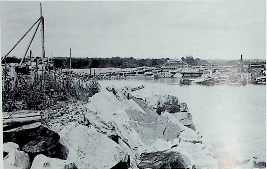
Buckhorn dam and bridge of squared lumber with rock core. 1906. During the early phase of replacement with a new steel-reinforced concrete dam. N.B. Steam engine used during construction ( right ). (Courtesy Trent-Severn Waterway).
