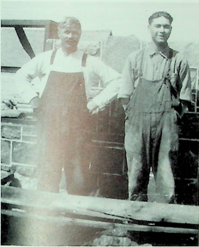
Henry Parker and son Harry building the barn wall for Bruce McKinty, now part of the Six Foot Bay golf clubhouse, 1923.
