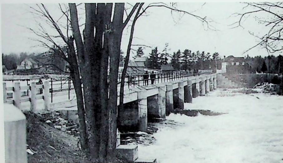
Reinforced concrete dam and single-lane bridge at Buckhorn, completed 1908. View to north, lockmaster's house ( right background on Harvey Township side ), existing bridge ( left of lockmaster's ), St. Matthew's Church ( left ). 1930s. (Courtesy Trent-Severn Waterway).
