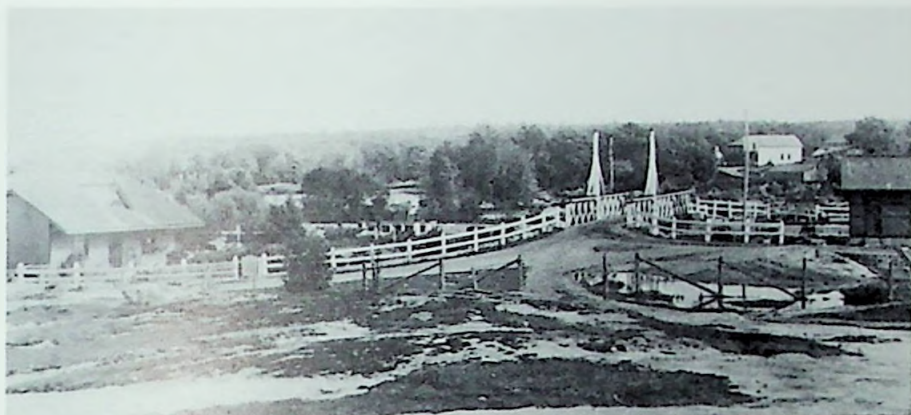
Buckhorn Lock from north, circa 1900. The 1888 timber swing bridge ( centre ), lock-master's house ( left ). Purser's store on the Smith Township side ( white building, right background ). (Courtesy Frank Cody, Buckhorn).
