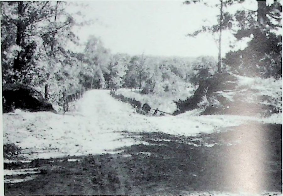
Government Road, southern section viewed to south, early 1920s.
