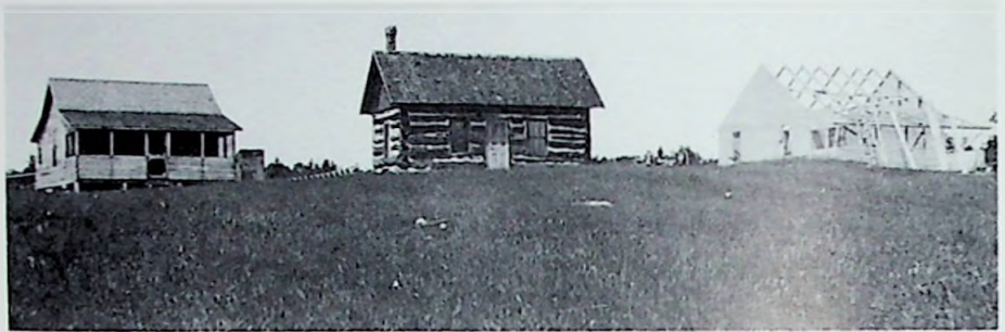
Cottages of varying ages at Scotsman's Point, 1934. In centre is an old squared-log house converted to cottage-use by visitors, left is a more recently-built cottage with typical verandah, and on right is a similar cottage under construction. (Courtesy Grace Smith)
