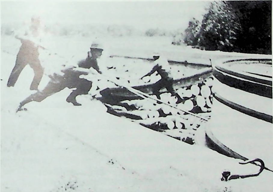
Blewett's river-drive, circa 1925, using pike-poles to position logs in Buckhorn Lock astern of the steam tug "Pearl".
